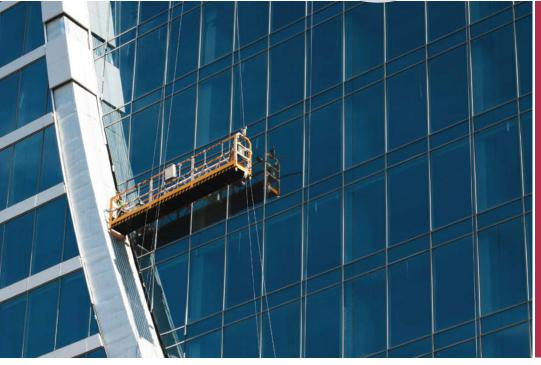
The innovative UpPro series man-riding traction hoists provide safe and reliable access for installation and maintenance of elevators, building facades, roofs, and more.
